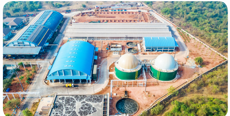
India's one of the finest Municipal Solid Waste Management Plants in Goa developed by SMC
