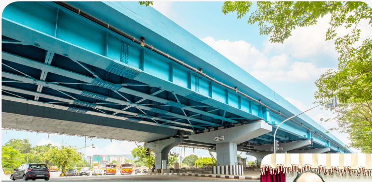
Southbound Flyover on EEH at AGLR Junction
